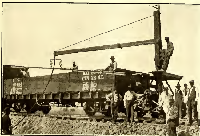
RAIL-LAYING PORTABLE CRANE USED ON KANKAKEE & URBANA TRACTION LINE
